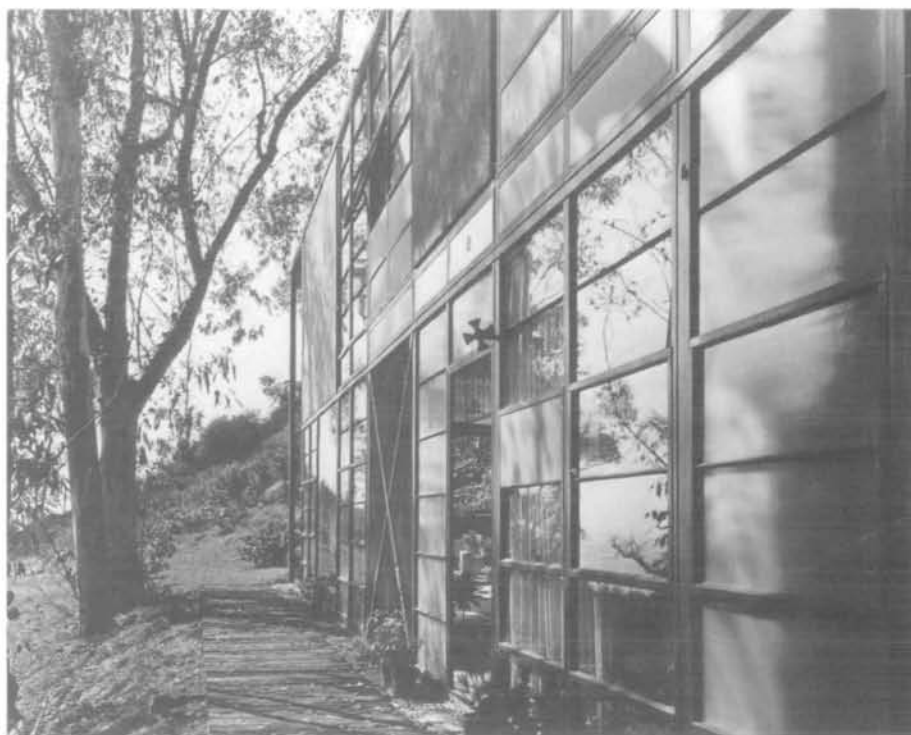
1 Front entrance, Eames House, Pacific Palisades, California, 1945–9
